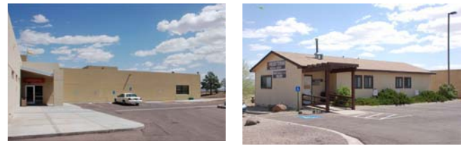
Fig. 2 Socorro General Hospital (left) and Surgery Office (right)
