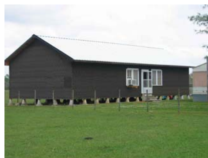
Fig. 3 Pier and beam, wood-frame structure
