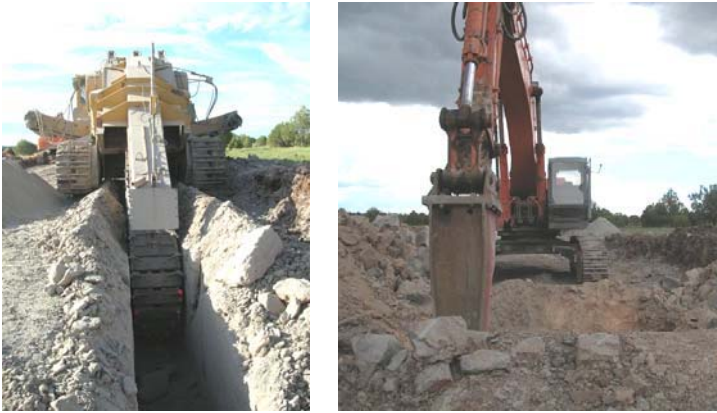
Fig. 1 Rock trencher (top) and impactor (bottom)
