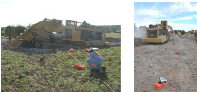
Fig. 2 Perpendicular (left) and parallel (right) arrays of seismographs towards the trencher
