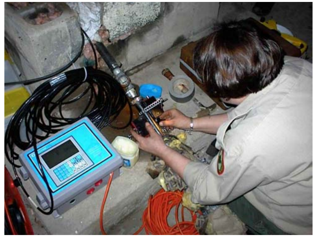
Measuring yield using ultrasonic flow meters
